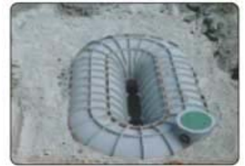
Step 4 Fill around perimeter of tank with backfill material.
