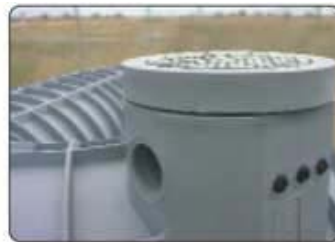
Step 7 Position adjustable collar if required. Note: Silicon must be used between the joint of tank inlet & the collar to form a water tight seal.
