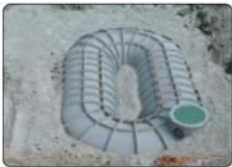
Step 5 Fill centre of tank with backfill material above the halfway flange.
