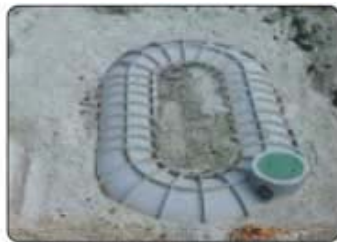
Step 6 Fill centre of tank with backfill material and/or concrete ballast. For details see "T:/BrochPDF/Watertanks/Tankmasta/Underground Tanks-Installation_8pg_np" available on request
