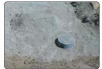
Step 8 Tank is now ready to be covered and landscaped over.
