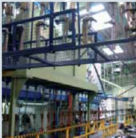
Powder coating unit
