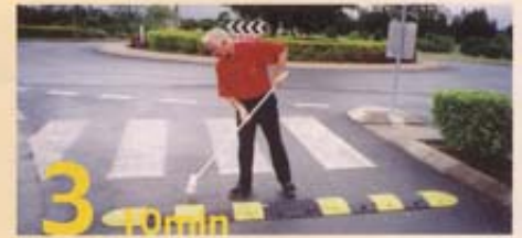
3 10min Final check-pack up and clean site
