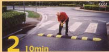
2 10min Drill holes and insert fasteners
