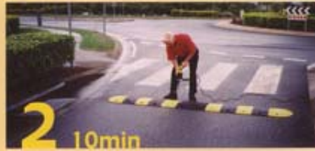
2 10min Drill holes and insert fasteners
