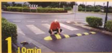
1 10min Check location, measure and position speed hump
