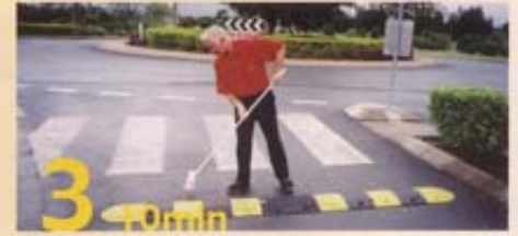
3 10min Final check-pack up and clean site
