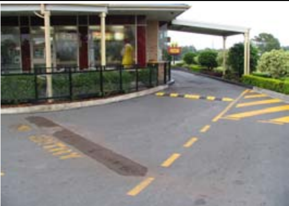
McDonalds Metal replacement
