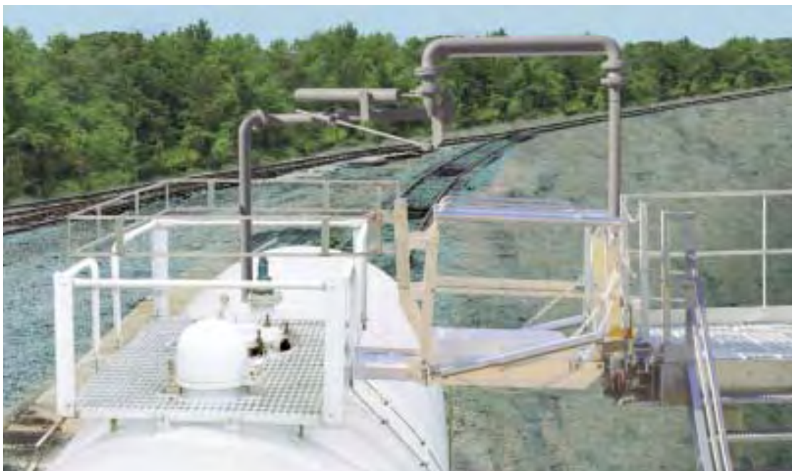
Optional 42" handrail meets OSHA requirements. Swivel mounted gangway reduces spotting problems.
