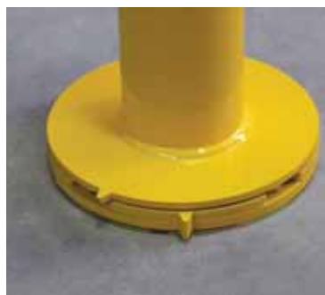
Bollard installed into shoe.
