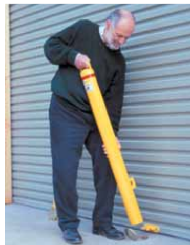
Insert-twist-lock.
